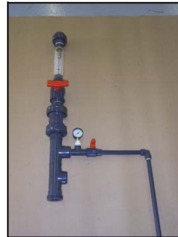
Discharge Piping Assembly
